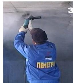
Make U-shaped indents along the whole length of the cracks, seams, joints, couplings and junctions and around all service line entries. Clean the indents with a wire brush. Remove the loose concrete layer (if any). Using a jackhammer, rout out the cavities of the pressure leaks to a width of 25 mm or more and to a depth of 50 mm or more, making them wider towards the interior (if possible, in the shape of a dovetail). Remove the loose, peeled off concrete from the inside of the leak.
